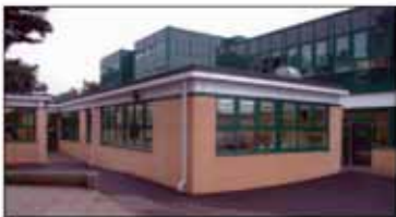
Recently completed Les Quennevais School SEN extension
